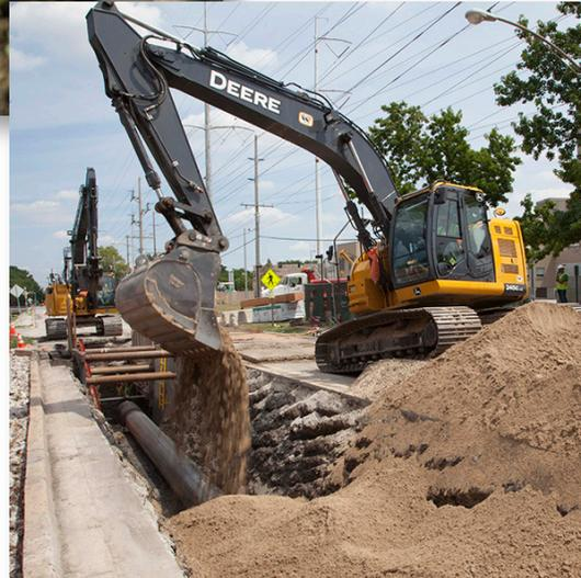
◀ NPL installed 3.5 miles of 24" steel pipe. The project included construction of three transmission stations and the destruction of one; three HDD bore shots under a railroad, river and stream, totaling 3000 feet; hydrostatic testing of all the mainline; and 100% restoration.
